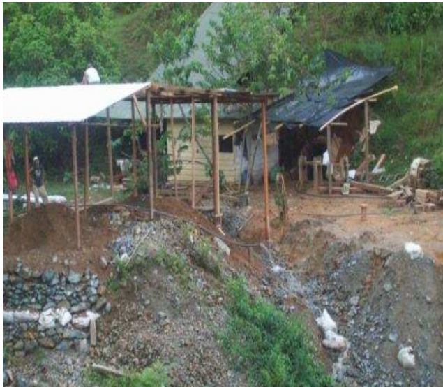
OVERVIEW OF THE FIRST TUNNEL NEXT TO THE OFFICE AND NEW TUNNEL! A HOUSING STRUCTURE FOR THE WINCH, VENTILATOR AND NEW TUNNEL IS BEING CONSTRUCTED. A SIDE VIEW OF THE NEW 60° TUNNEL ENTRANCE 2010.
