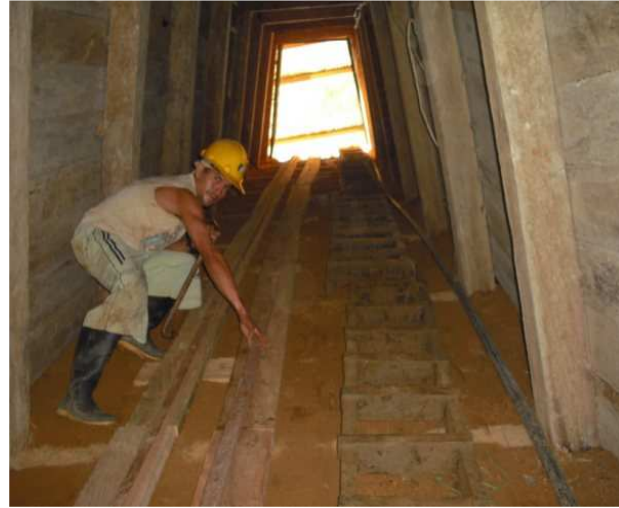
INSIDE NEW 60° TUNNEL WORKERS BUILD THE WOODEN BASE FOR THE STEEL RAILS. THESE RAILS WILL BE USED TO HAUL ORE CARTS UP WITH THE WINCH AND PULLEY SYSTEM SET UP OUT SIDE THE TUNNEL.
