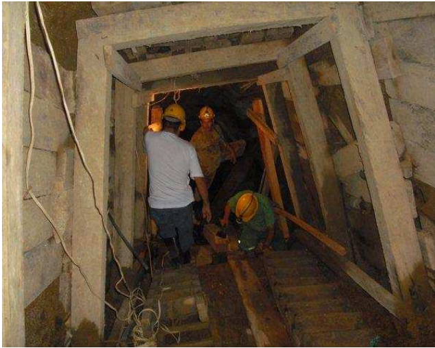
INSIDE NEW 60° TUNNEL WORKERS BUILD THE WOODEN BASE FOR THE STEEL RAILS. THESE RAILS WILL BE USED TO HAUL ORE CARTS UP WITH THE WINCH AND PULLEY SYSTEM SET UP OUT SIDE THE TUNNEL.
