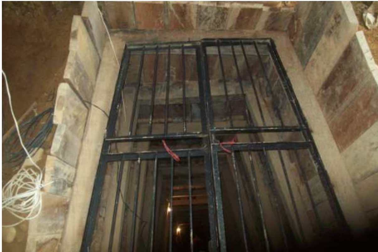
POWDER STORAGE UNIT AT MINE #4395 LAS PALMERAS JANUARY 2010 WITH FENCE AND GATE INSTALLED. STEEL GATES HAVE BEEN INSTALLED AT THE MINE ENTRANCE FOR SECURITY REASONS AND SAFETY ISSUES.
