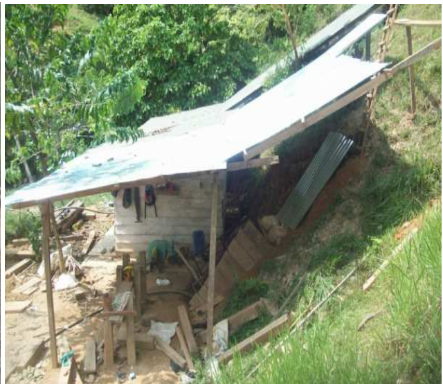
OVERVIEW OF THE FIRST TUNNEL NEXT TO THE OFFICE AND NEW TUNNEL! A HOUSING STRUCTURE FOR THE WINCH, VENTILATOR AND NEW TUNNEL IS BEING CONSTRUCTED. A SIDE VIEW OF THE NEW 60° TUNNEL ENTRANCE 2010.
