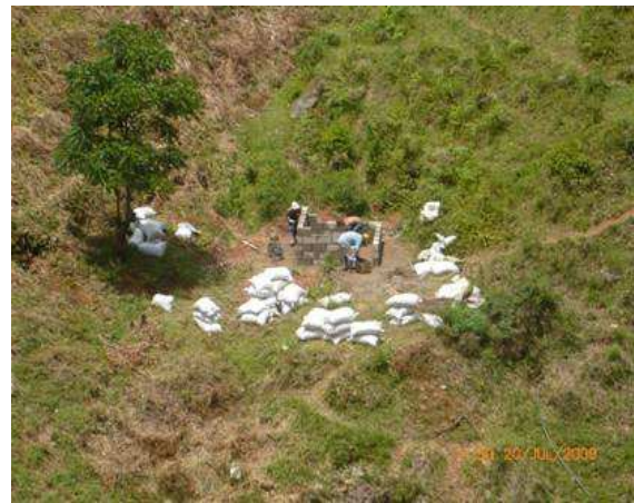
The worker standing in front of the cinder blocks is currently building the room to store explosives and tools. He is also under contract to build a cement floor for the office and tool shed.
