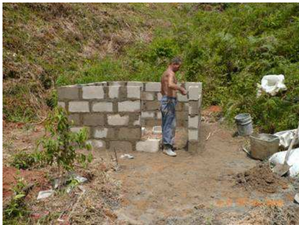
The worker standing in front of the cinder blocks is currently building the room to store explosives and tools. He is also under contract to build a cement floor for the office and tool shed.
