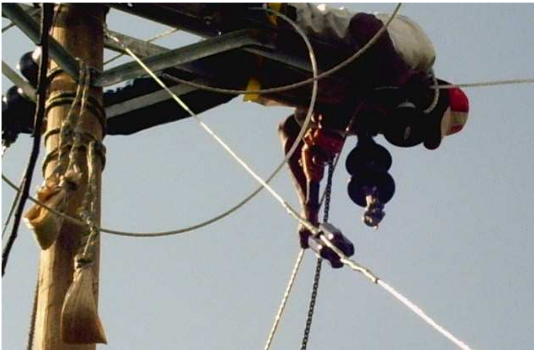
WORKERS ARE ON TOP OF THE POLE WITHOUT ANY HEAVY EQUIPMENT.
