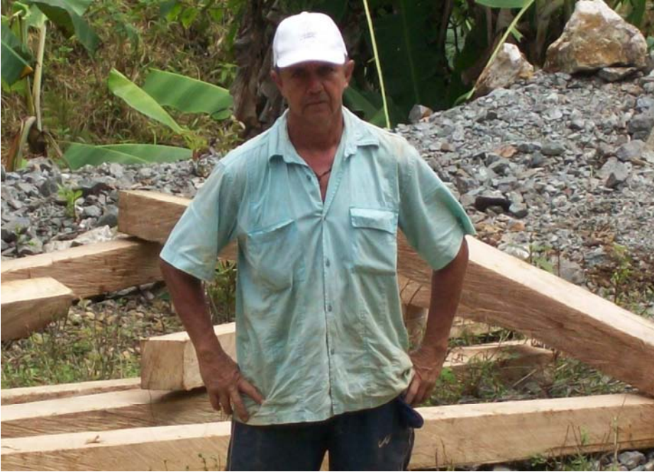
ON SITE MANAGER WITH 6" x 6" x 10' LUMBER AT THE LAS PALMERAS MINE SITE THAT WAS BROUGHT IN 600 METERS FROM THE ROAD.
